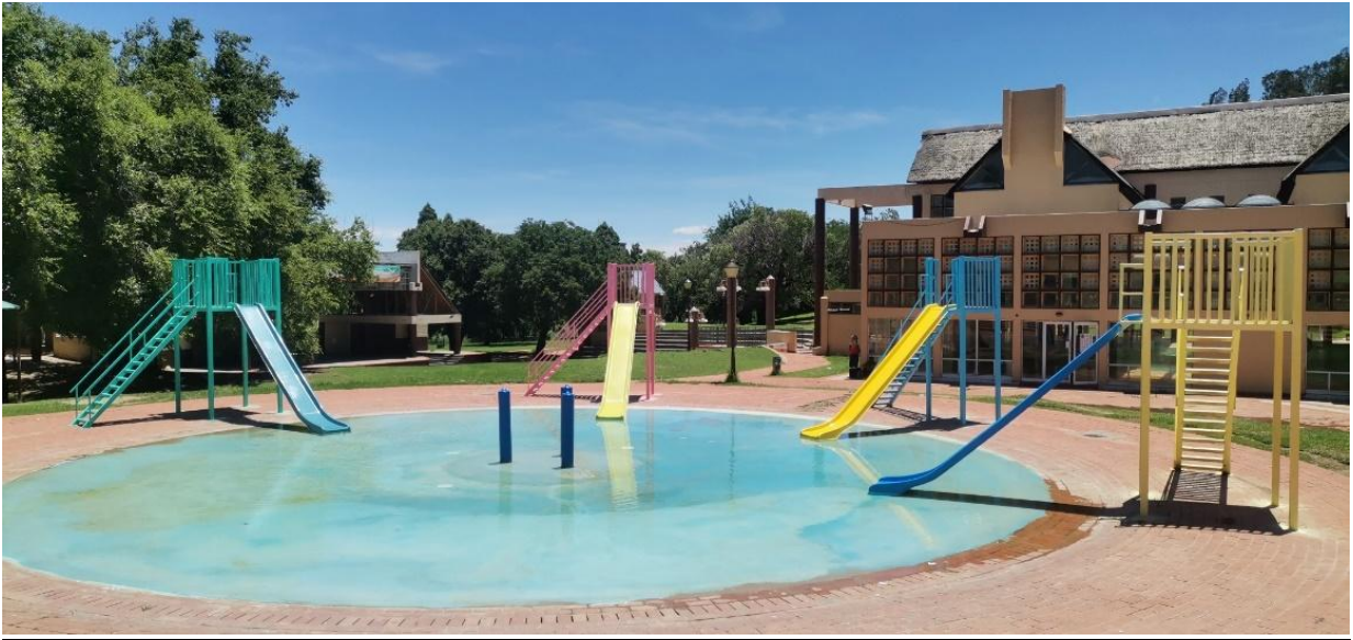
Installation of New water slides
