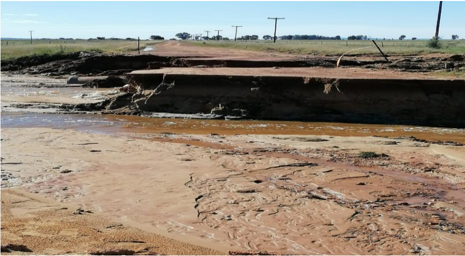
Figure 6 Eroded Road
